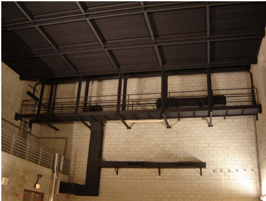
Ceiling of Stage Area Stage Grid has already been installed.
