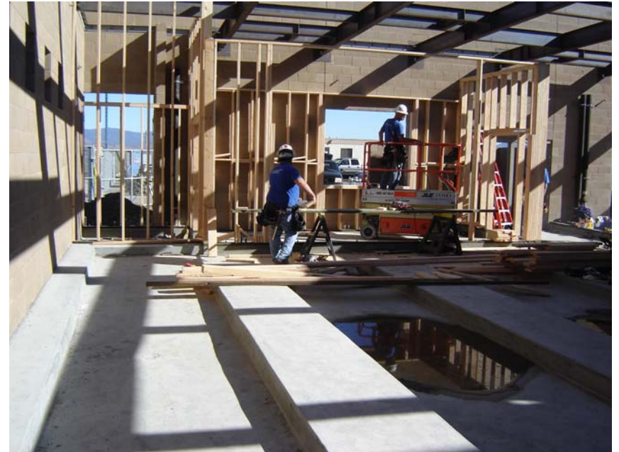
Wood Framing in Locker Rooms
