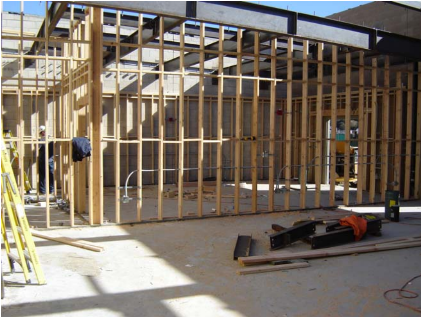
Wood Framing in Classrooms
