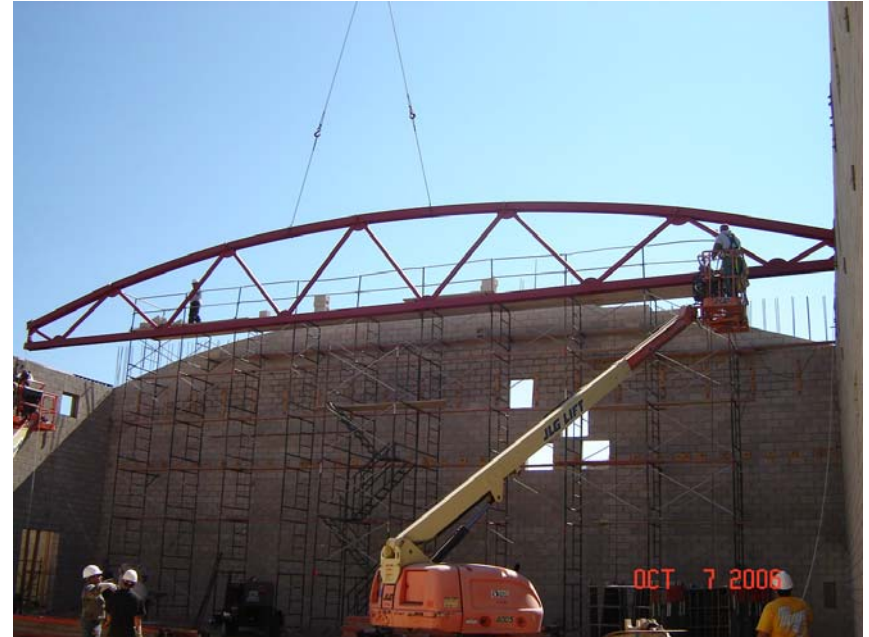
Gymnasium Roof Trusses Trusses span a distance of 80 feet.
