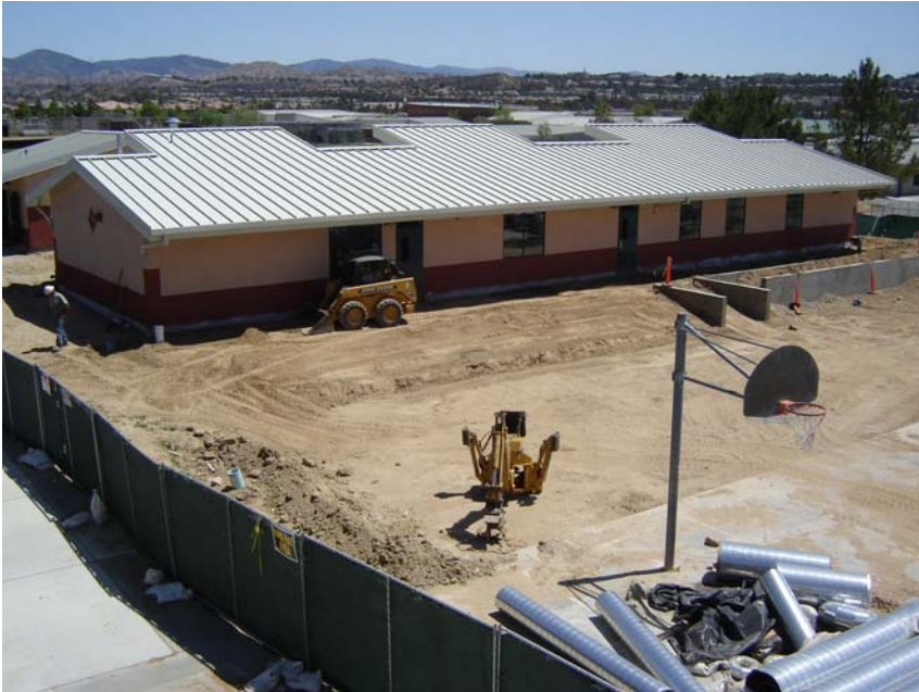
Building Exterior nearly complete
