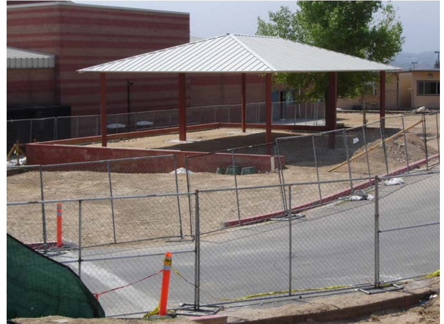
Shade Structure in-place
