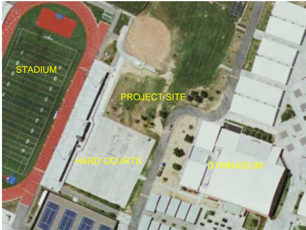
Site Prior to Construction
