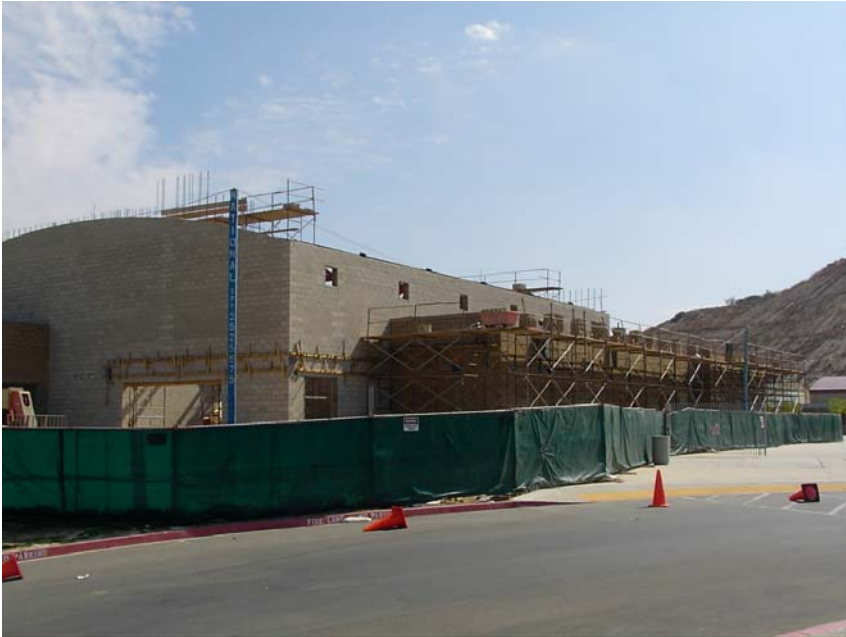
Masonry Walls Being Completed September 2006
